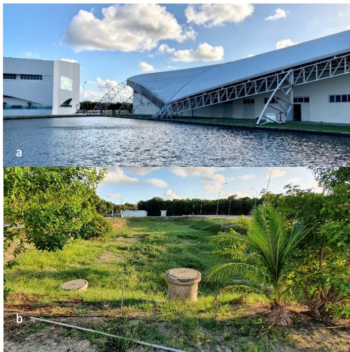
Figure 12. Convention Centre of Joao Pessoa: a) Large roofs with deco ponds; b) infiltration system
