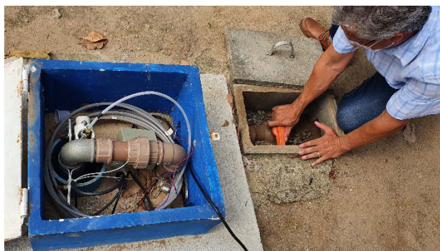
Figure 11. SMART-Control pilot site in Joao Pessoa: starting the infiltration
